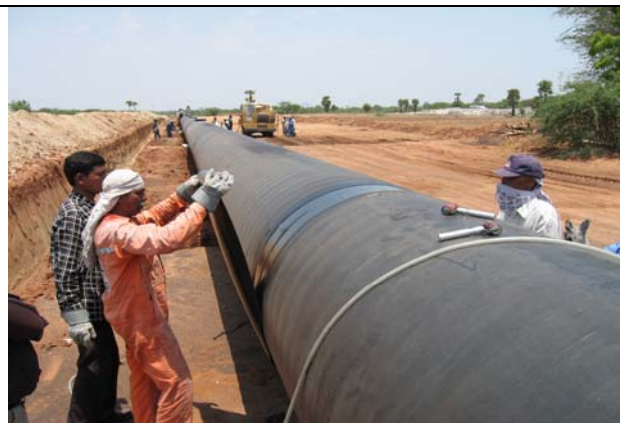
印度东气西输管道工程防腐补口 India East to West Gas Pipeline Joint Coating
