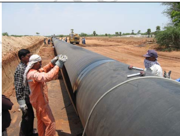
印度东气西输管道工程防腐补口 India East to West Gas Pipeline Joint Coating
